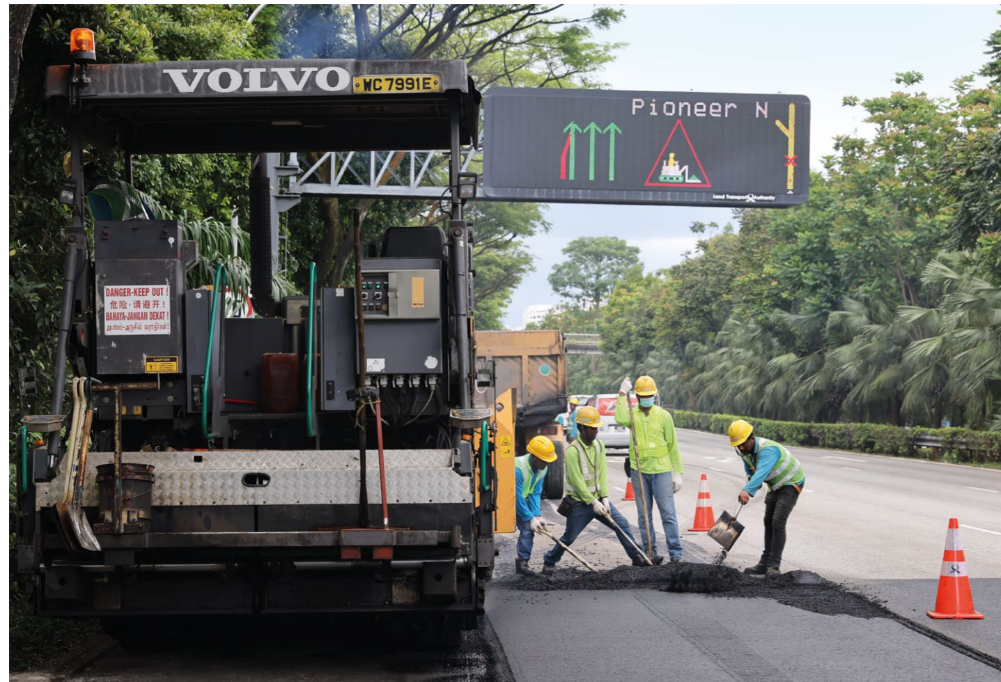
Researching the use of plastic waste in asphalt roads. – Paving Green Roads, Singapore
