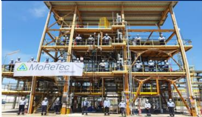
MoReTec Pilot Plant, Ferrara, Italy
